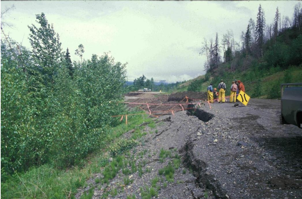
**Figure 7: A reactivated slump earth flow after an up-grade of the Morice Road. Attempts to stabilize the road have cost millions of dollars over the past 30 years.**
